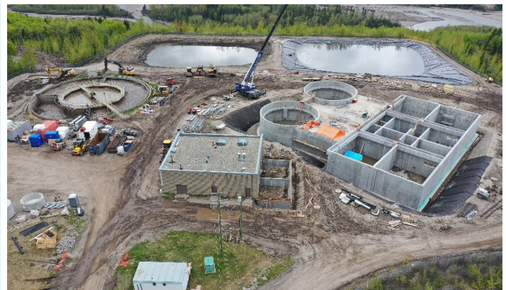
Aerial view of the new Wastewater Treatment Plant.
