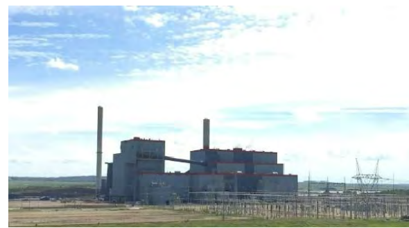
Electric Power Generation
