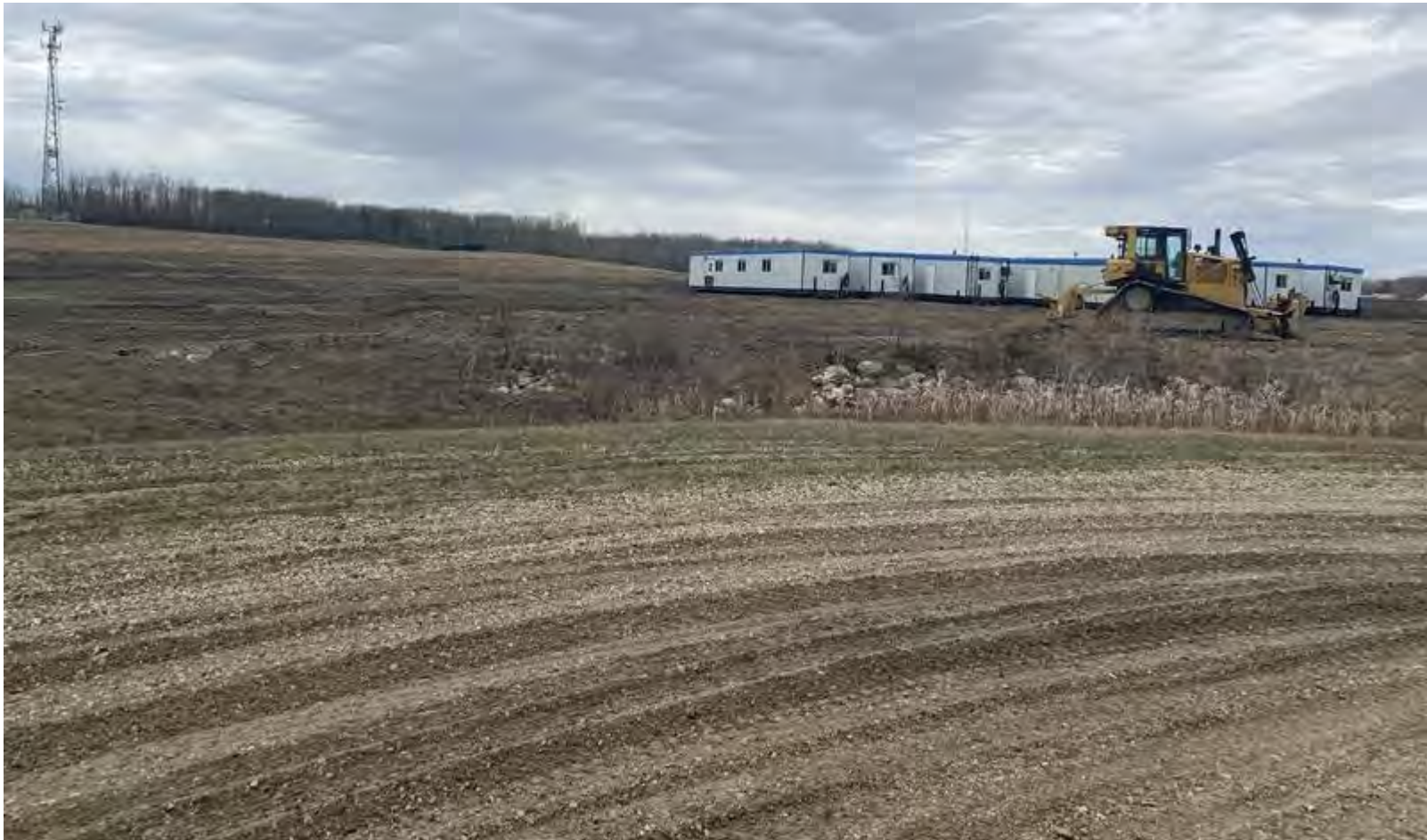
East Lot Boundary at Traffic Bulb facing NW
