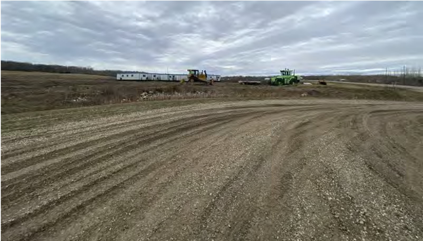
East Lot Boundary at Traffic Bulb facing North
