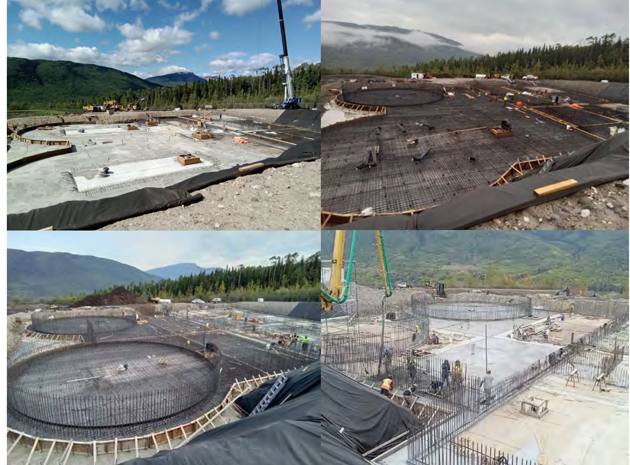
Mudslab and Base Slab
