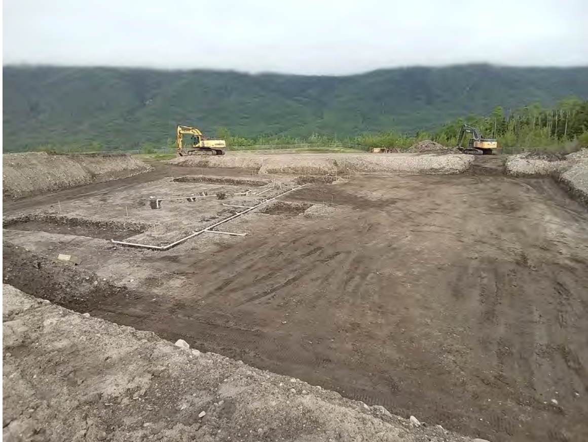
Subgrade Excavation and Under Slab Utilities
