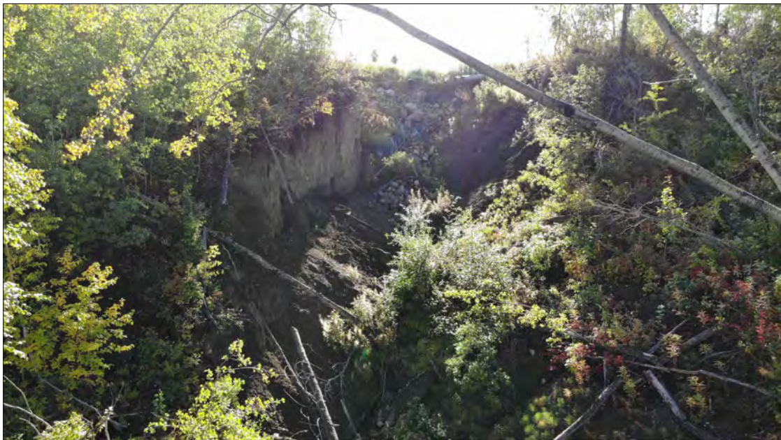
PHOTO 4 -SCOUR CHANNEL, LOOKING EAST, RANGE ROAD 205 IN DISTANCE; NEAR-VERTICAL ERODED FACES, LOOSE TALUS PILES IN CHANNEL, FALLEN TREES
