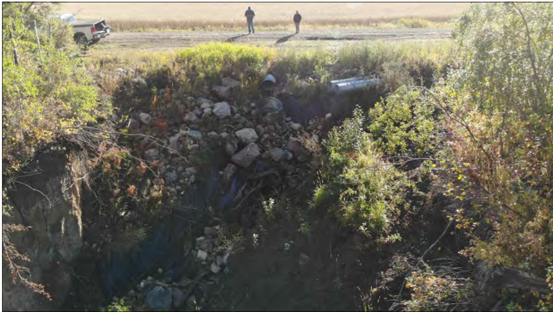
PHOTO 3 - RANGE ROAD 205 AT BEGINNING OF SCOUR CHANNEL, LOOKING EAST; CULVERTS DIRECTING RUNOFF INTO CHANNEL, EXPOSED GEOTEXTILE, LOOSE COBBLES, BOULDER AND GRAVEL FILL
