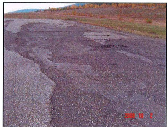
Severe Ravelling and Asphalt Failure – Runway 08-26 Turnbays
