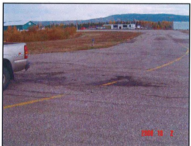
Severe Ravelling and Asphalt Failure – Taxiway “A”
