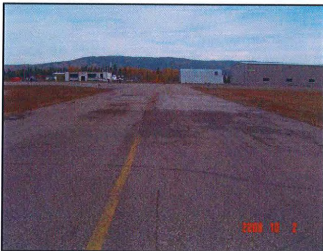
Severe Ravelling and Asphalt Failure – Taxiway “A”
