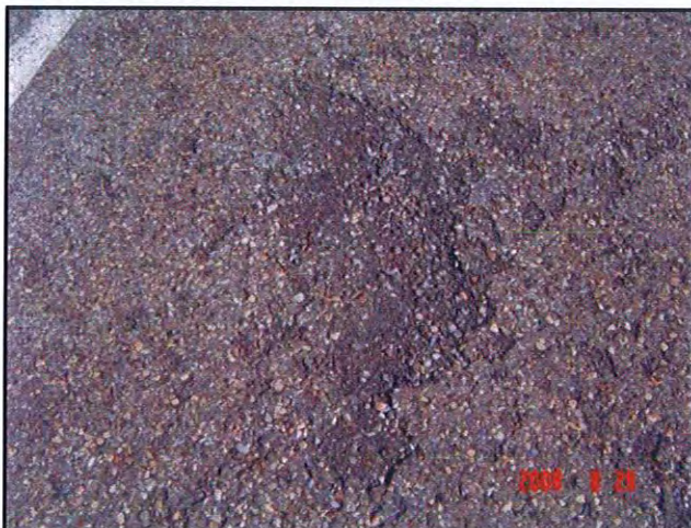
Severe Ravelling and Asphalt Failure – Runway 08-26
