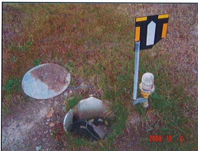
Deteriorated Edge Lights
