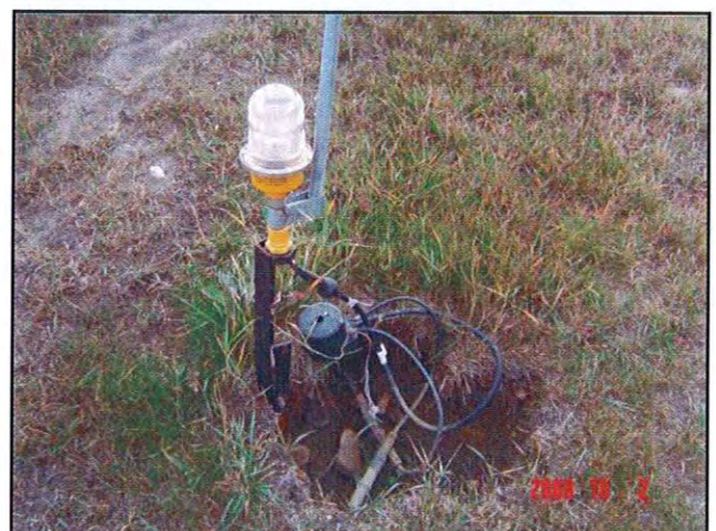
Deteriorated Edge Lights
