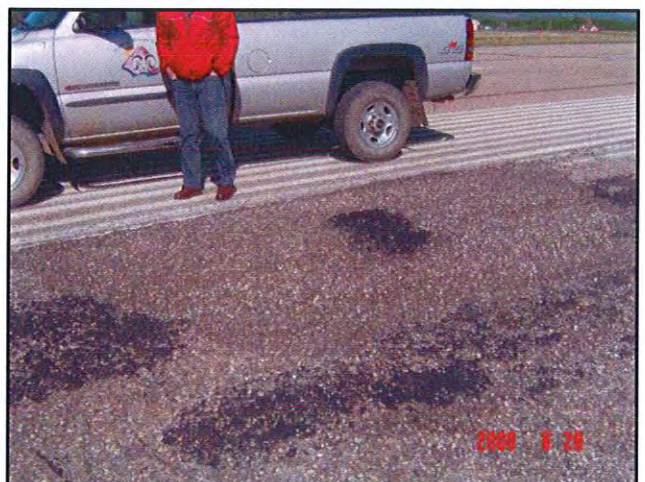
Severe Ravelling and Asphalt Failure – Runway 08-26
