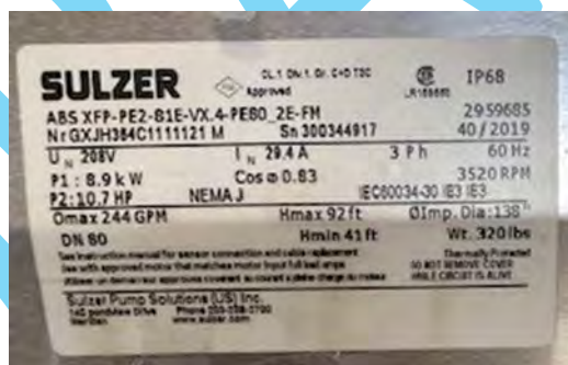
Ridgevalley Lift Station Pump Tag
