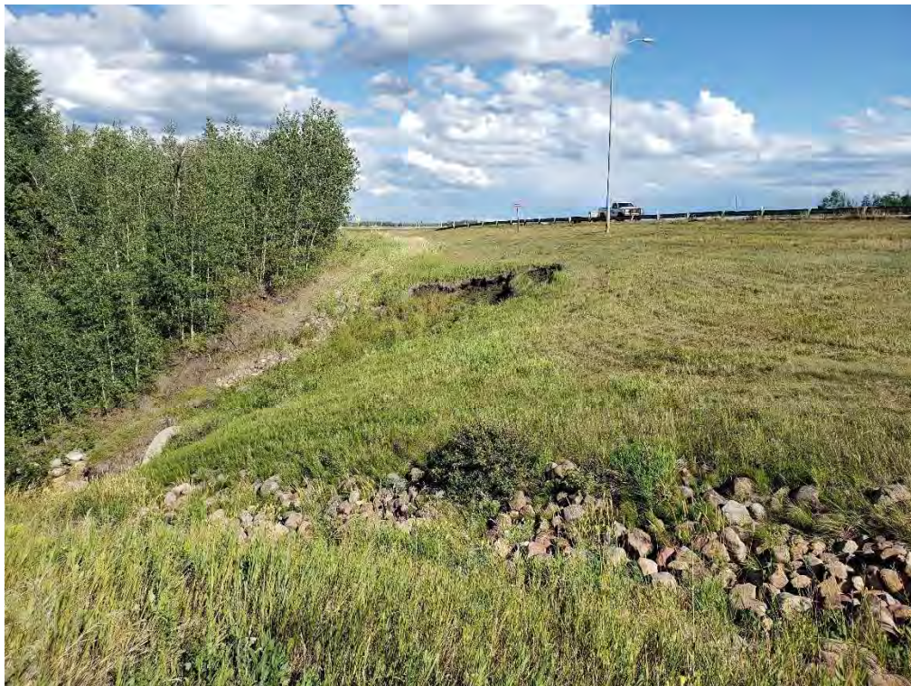
Photo 6 – Landslide below Highway 43 in embankment fill
