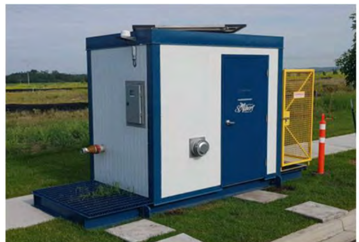
Insert 5-1: Typical Bottle Fill Station
