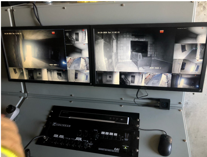
Example of control center
