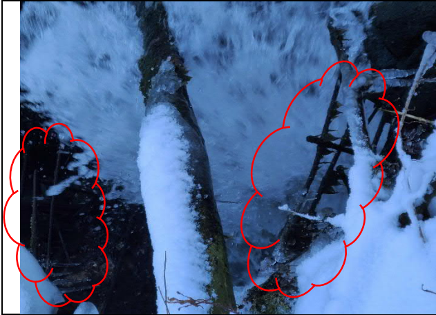
Outfall Structure – Exposed Rebar
