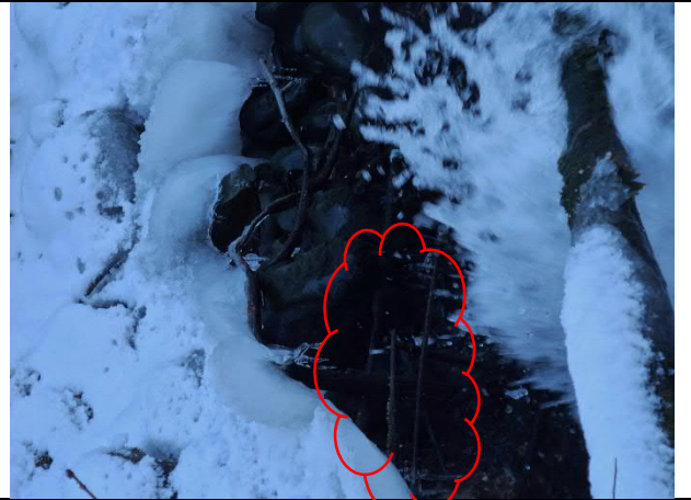
Outfall Structure – Exposed Rebar
