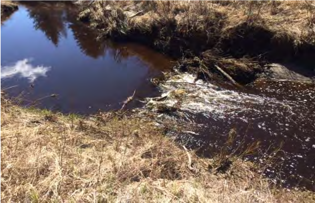
Photo 6. Showing the remnants of dam 1 prior to removal on May 16, 2020
