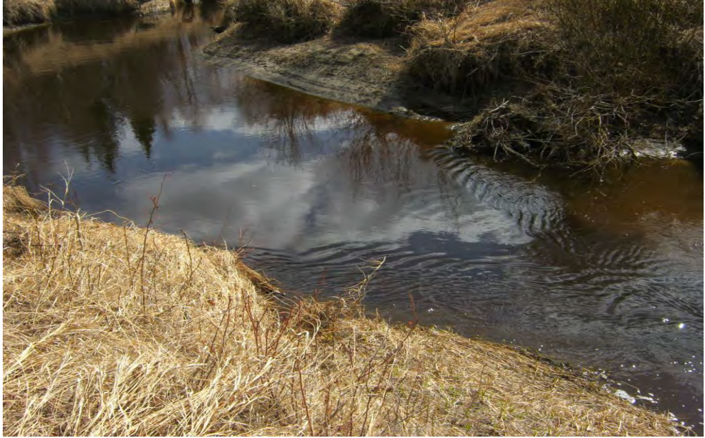
Photo 6. Showing dam 1 following removal of debris on May 16, 2020
