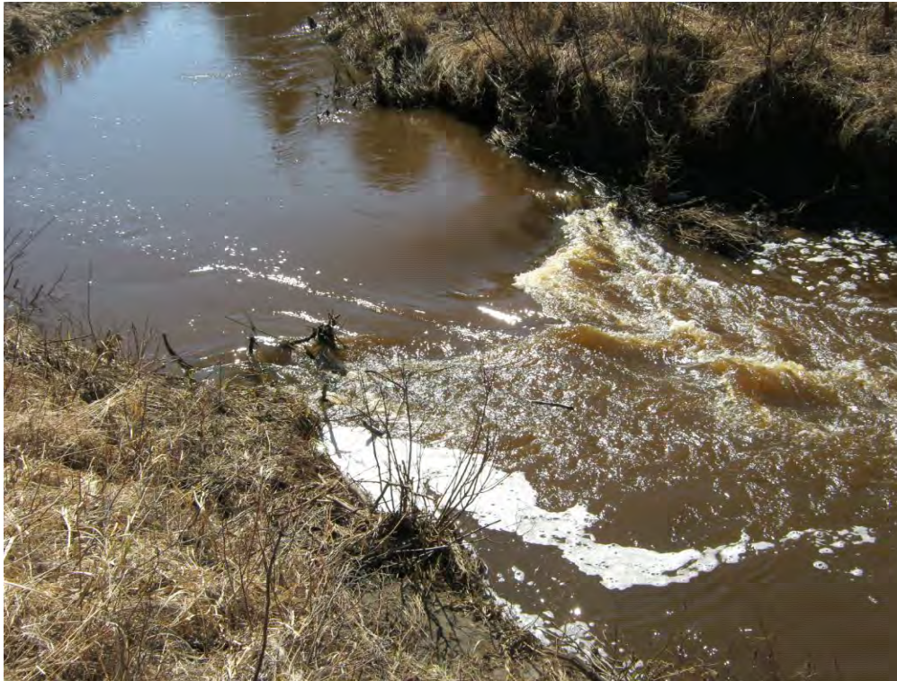
Photo 2. Showing Dam 1 on May 2, 2020
