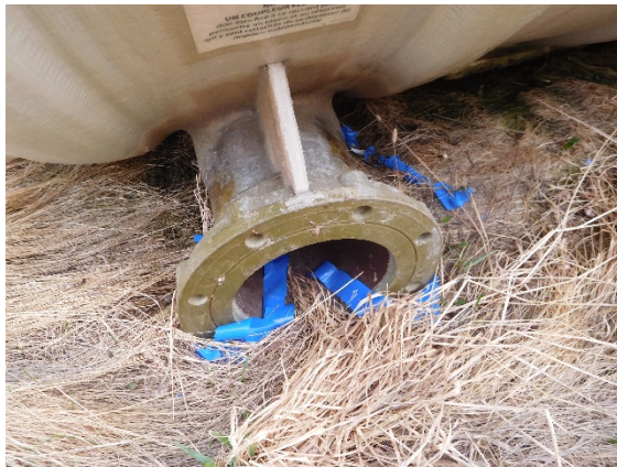
Figure 3: Restricted Flange Condition
