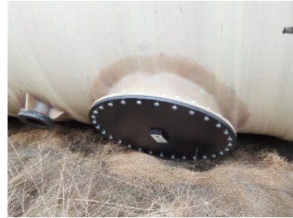
Figure 2: Manway with Blind Flange
