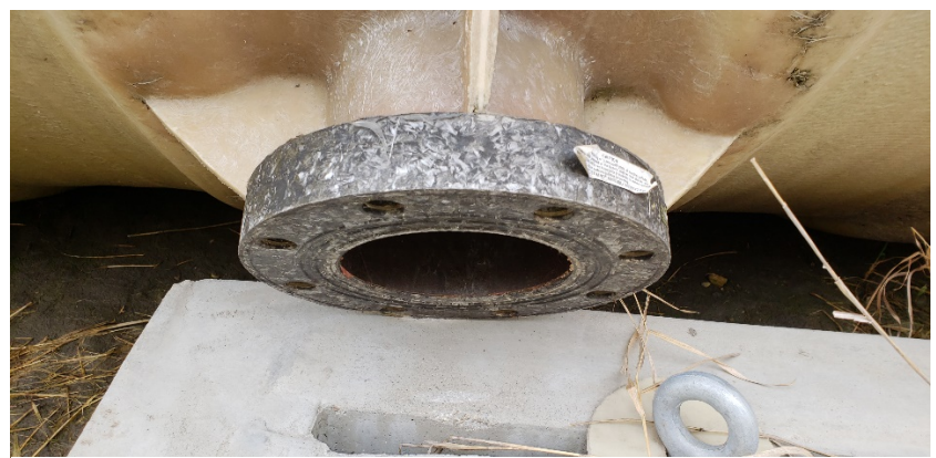
Figure 4: Flange Resting on Concrete Form
