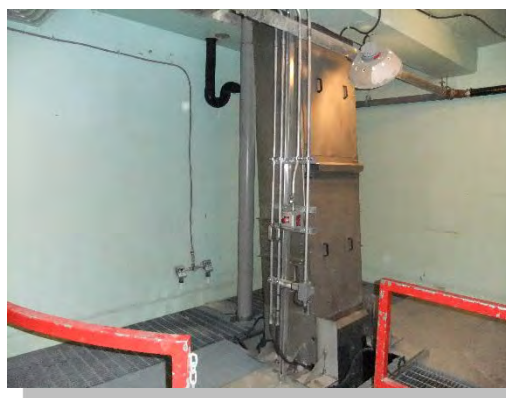
Influent Channel Screen Retrofit High River, AB
