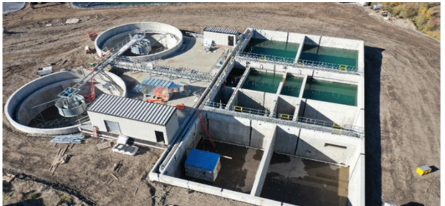
Figure 1 Clarifier X 2 and bio reactors
