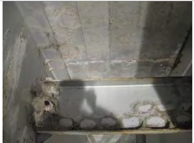
Photo 14: Swallow nests on diaphragm
