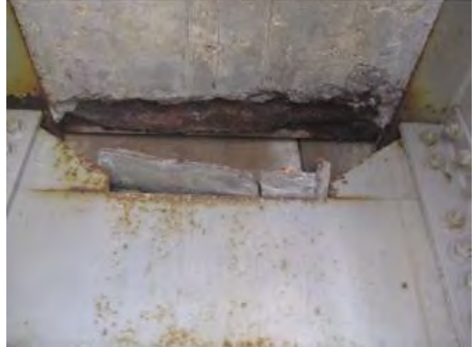
Photo 18: Spalling concrete at Pier 5 joint between Girders 2 & 3.
