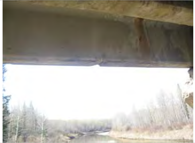
Photo 42: Damage to Girder 5, Span 6
