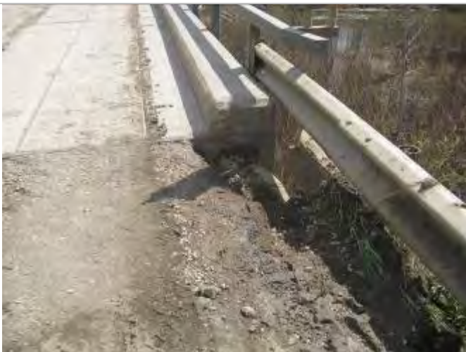
Photo 3: Wash out at S corner of W abutment (note step in approach rail to curb transition)
