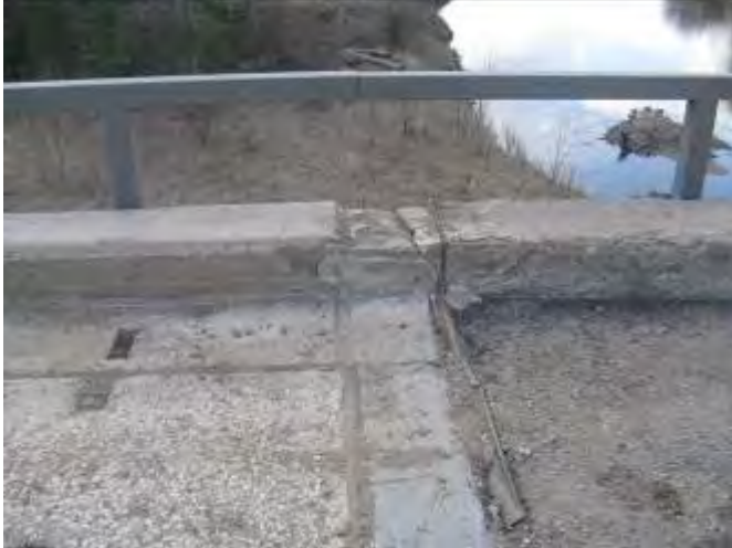
Photo 13: South curb joint Pier 5
