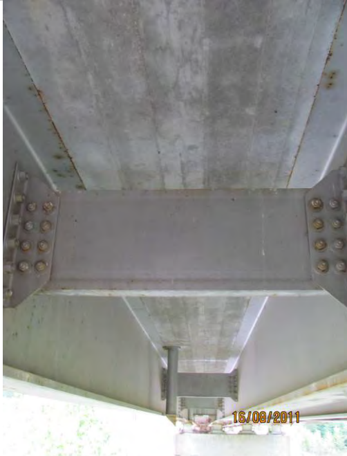
Photo 7: Condition of underside of principal spans appears to be little changed since last inspection.
