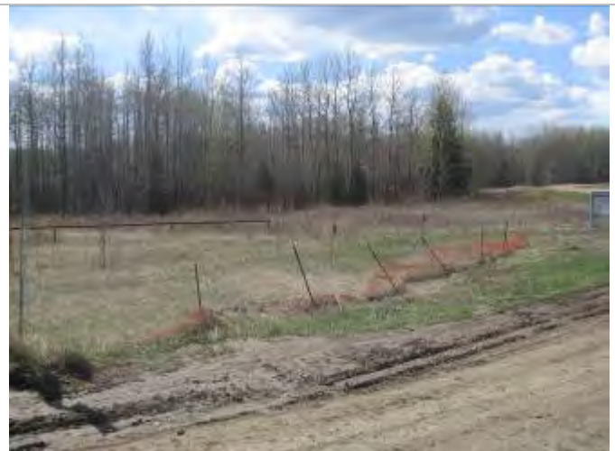
Photo 4: Buried gas line marked at SW approach
