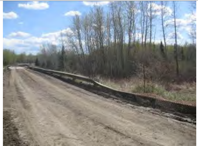
Photo 2: Damaged guardrail at SW approach
