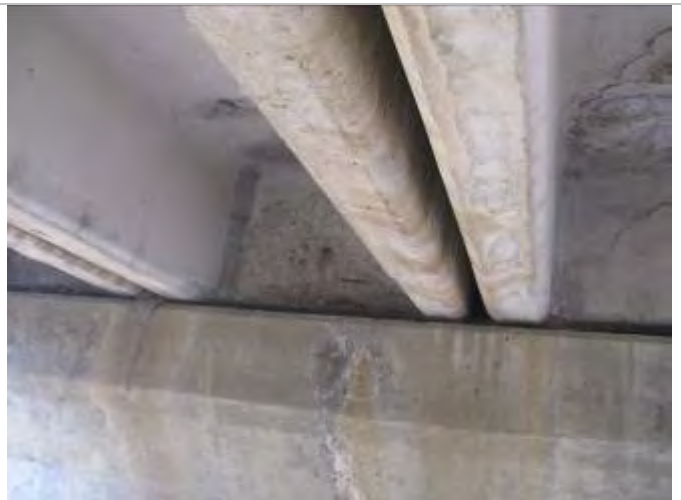
Photo 40: Spall on Girder 4 at Pier 5
