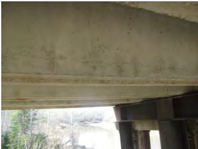
Photo 43: Longitudinal Crack in Girder 2, Span 7
