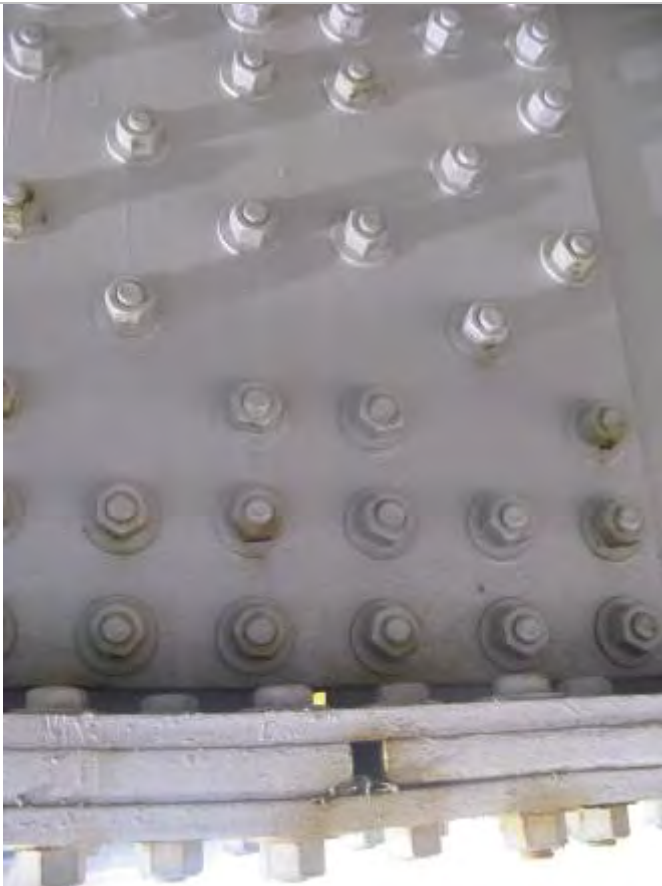
Photo 15: Distorted splice cover plate – Girder 3
