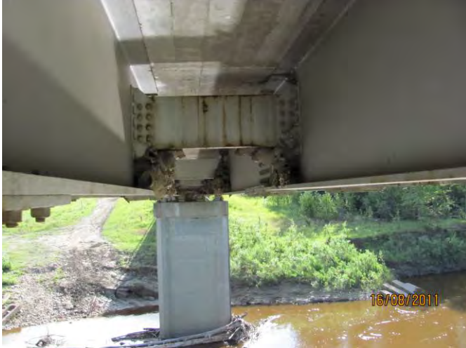
Photo 11: Main span. Bird nests around diaphragms.
