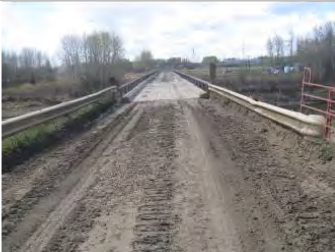
Photo 7: Transition of eastern approach rail to curb. Damage to NE approach rail.
