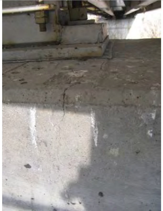
Photo 54: Cracking in Pier 3 piercap
