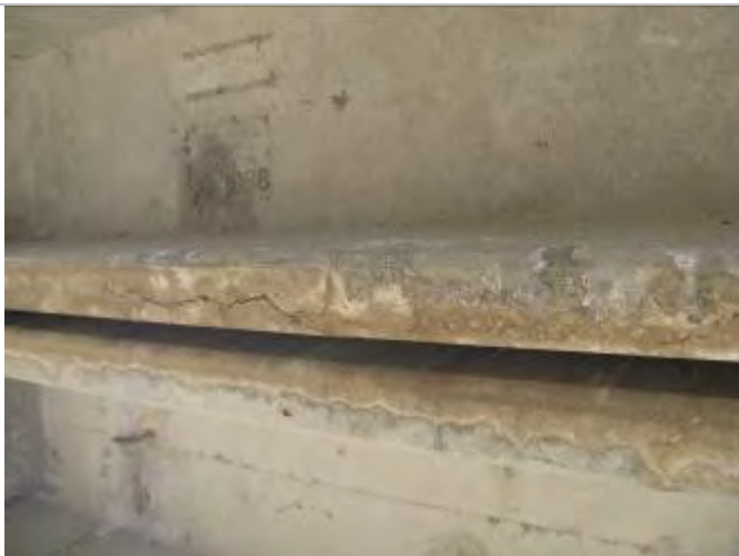
Photo 35: Wide crack in leg of Girder 2, Span 2
