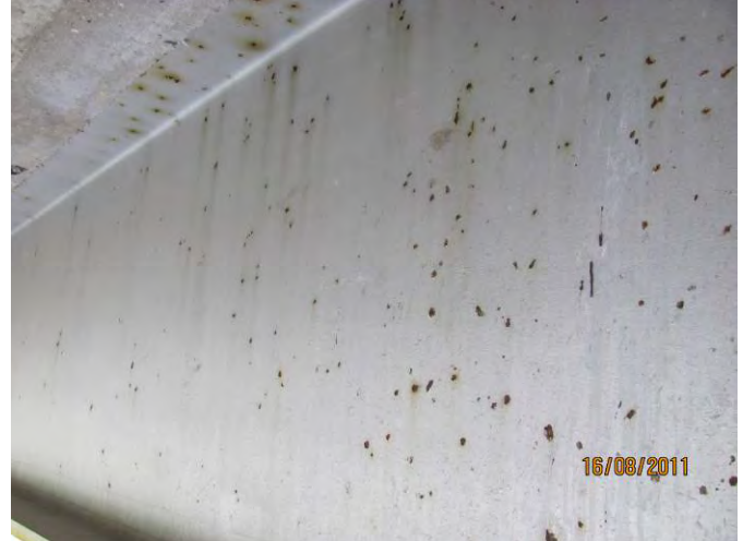
Photo 12: Some rust spotting of coating (approx.. mid span of main span)
