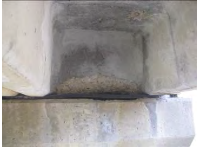
Photo 38: Spall on Girder 1 at Pier 5
