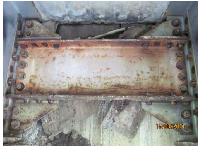
Photo 6: Diaphragm at Pier 2. Missing bolts and failing coating. Joint material falling through joint.
