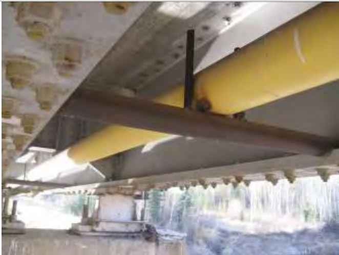
Photo 17: Honeycombing on underside of deck
