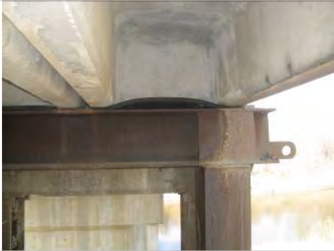
Photo 45: Deformed bearing, Span 7, Pier 6
