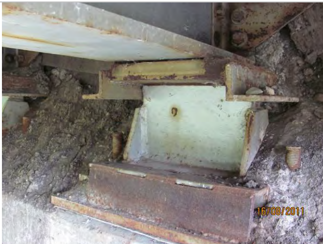
Photo 5: Debris on bearing shelf at Pier 2.
