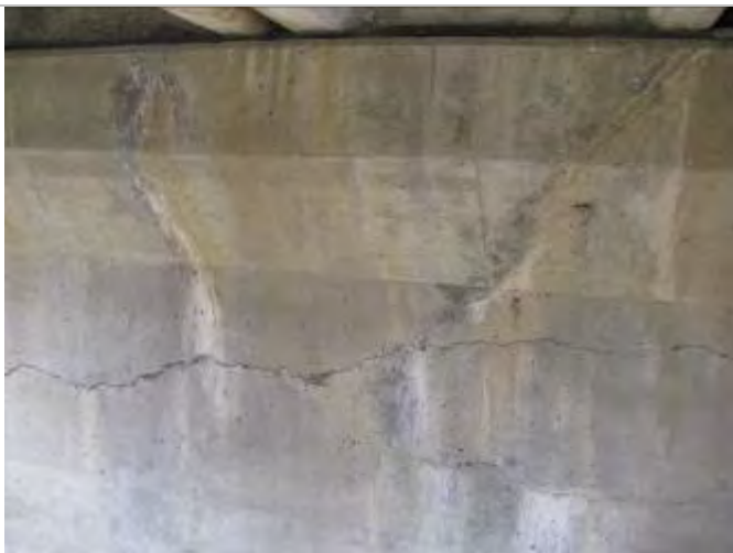
Photo 59: Wide crack in east face of Pier 5
