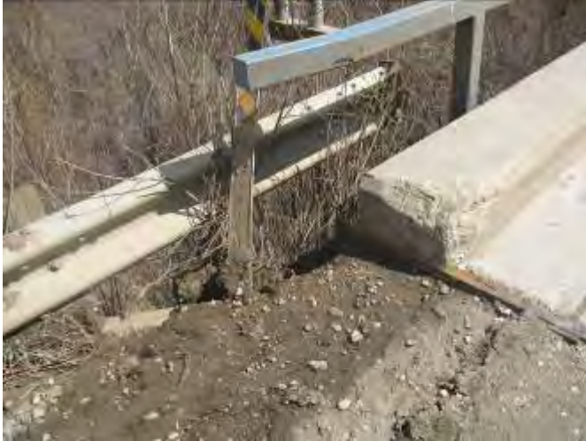
Photo 5: Transition of Approach Rail to curb at NW corner
