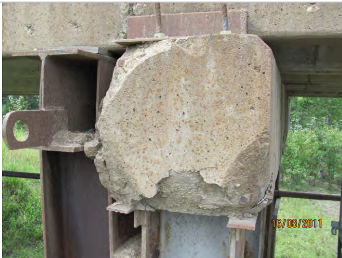
Photo 17: Pier 7 Spalling reinforcement
