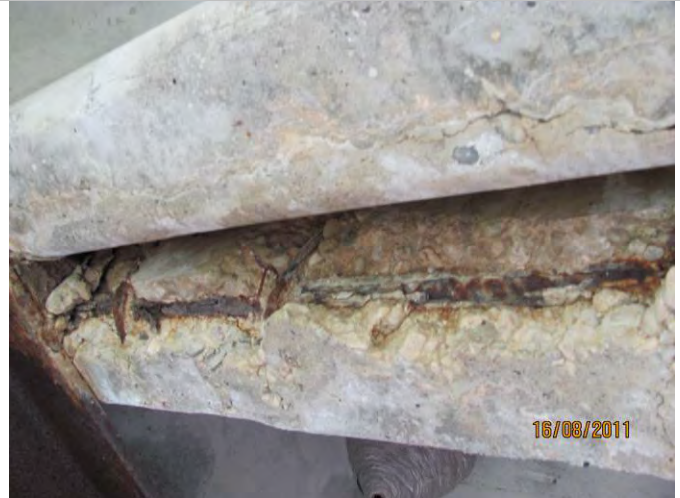
Photo 20: Gider D, Span 8 – spalled concrete and very corroded reinforcement
