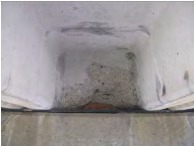
Photo 39: Large spall on Girder 2 at Pier 5
