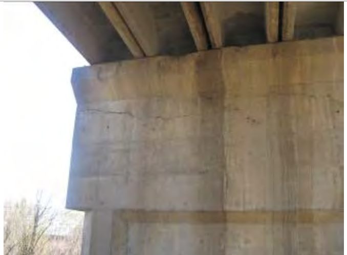
Photo 52: Crack in upstand wall of Pier 2
