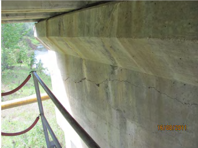
Photo 15: Wide crack in Pier 5
