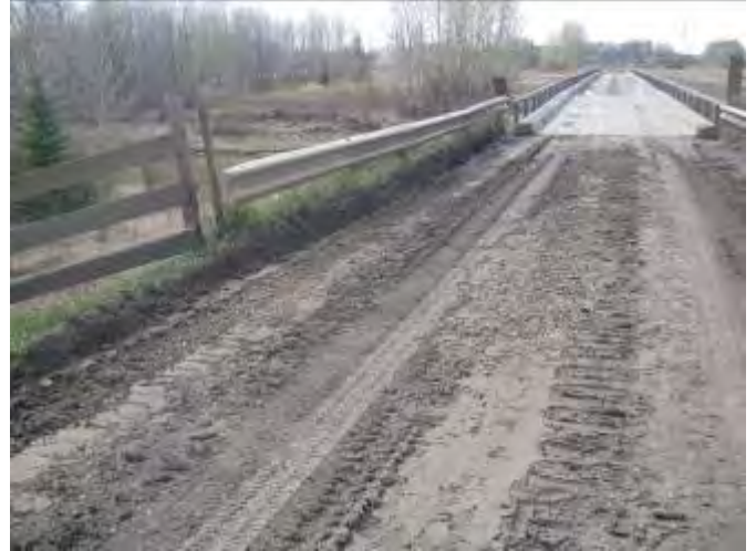
Photo 6: Lack of termination SE approach rail
