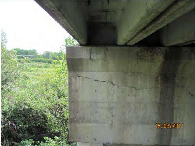
Photo 3: Very wide horizontal cracks in Pier 2.
