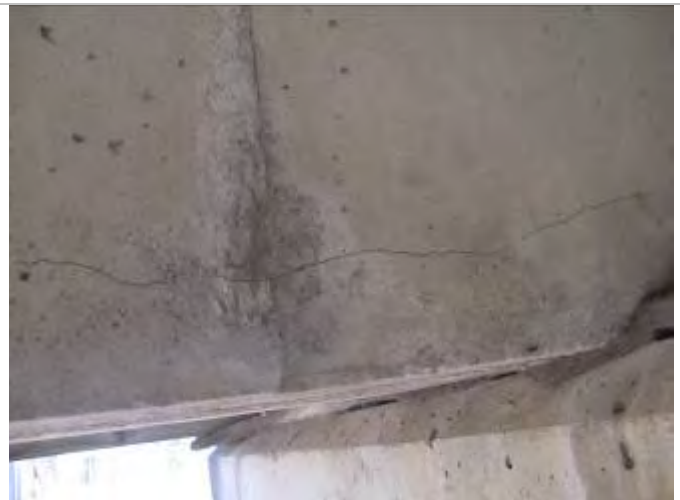
Photo 44: Cracked Girder, Span 7
