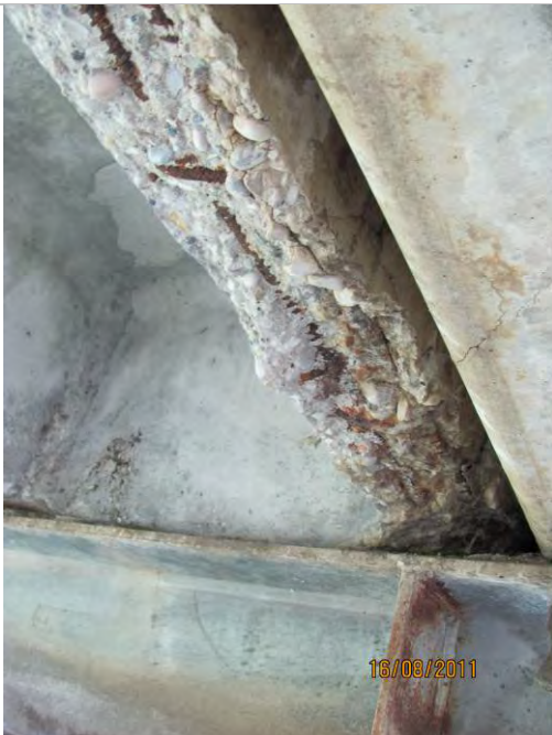
Photo 1: Girder D, Span 2 at Pier 1. Spalled concrete limits bearing of web on Piercap.
