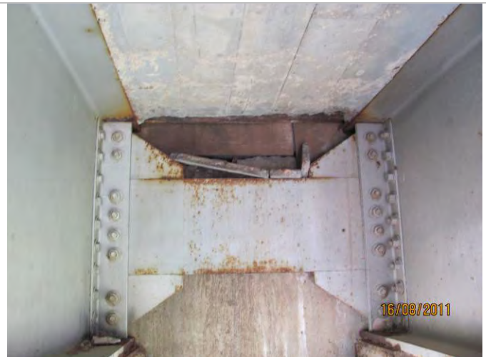
Photo 14: Corrosion of Diaphragm at Pier 3 and failing joint concrete
