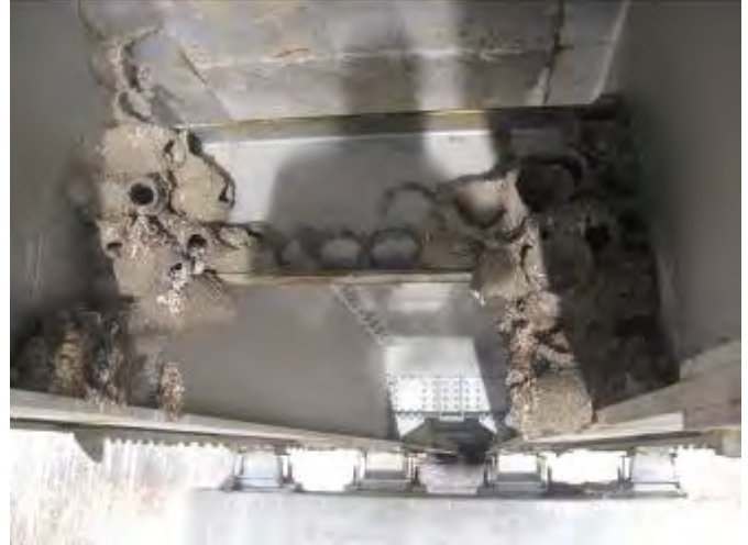
Photo 14: Swallow nests on diaphragm
