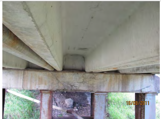
Photo 18: Pier 7 Deteriorating concrete
