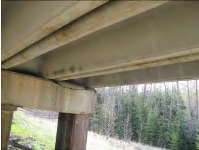
Photo 41: Crack in leg of Girder 4, Span 6
