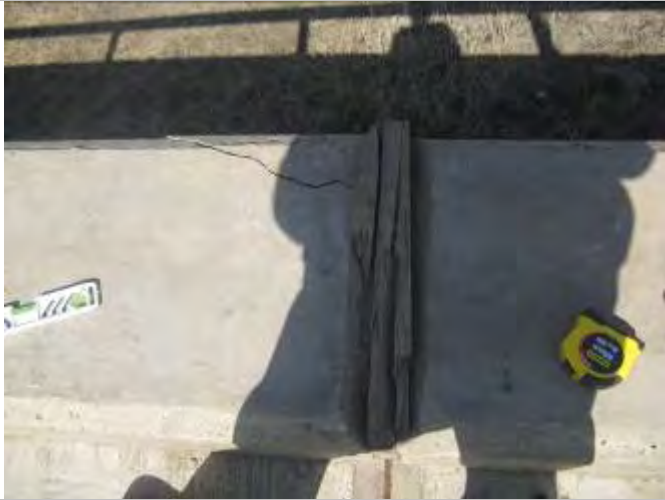
Photo 49: Cracked north curb, Pier 7
