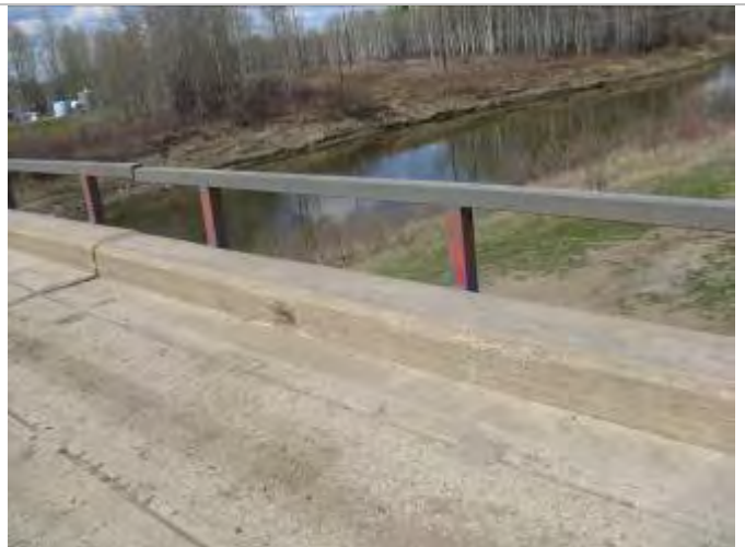
Photo 48: Spall in north curb of Span 7
