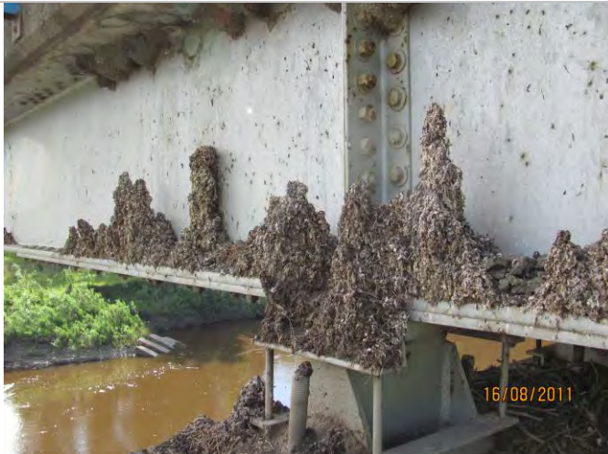
Photo 9: Debris on outside of girders at Pier 3.
