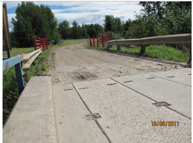
Photo 22: East approach with slight bump at end of bridge
