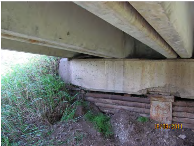
Photo 21: Spalled concrete at east abutment
