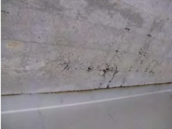
Photo 17: Honeycombing on underside of deck
