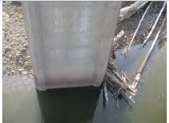
Photo 56: Crack in west face of Pier 4 pier stem
