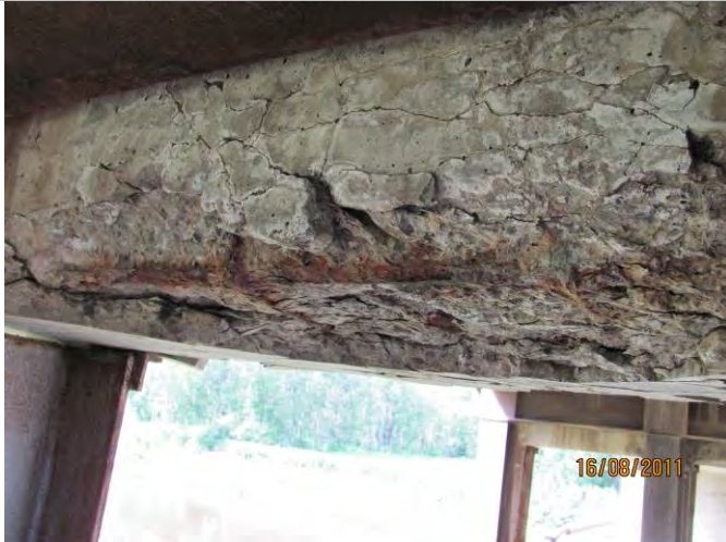
Photo 19: Pier 7 Spalled concrete and corroding reinforcement
