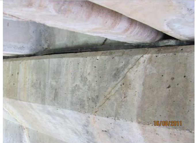
Photo 16: Diagonal crack in Piercap at Pier 5
