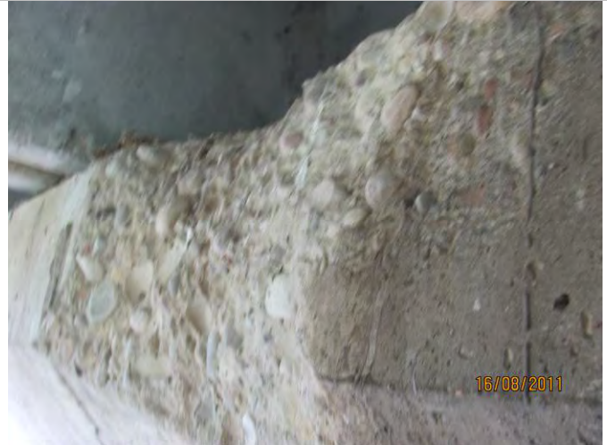
Photo 4: Spalling of Piercap at Pier 2.
