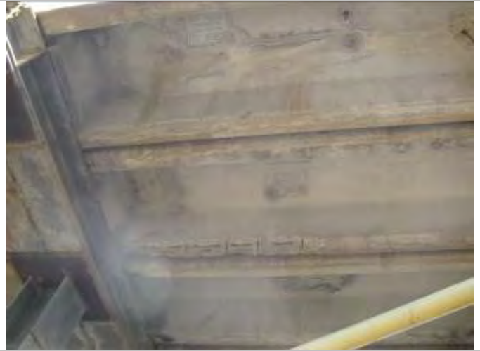
Photo 34: Spalling on Girder 2, Span 2
