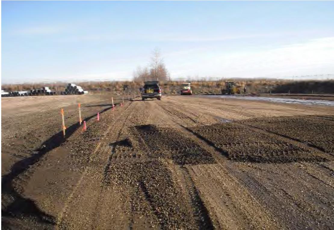
Granular Base Course Installation - Facing East
