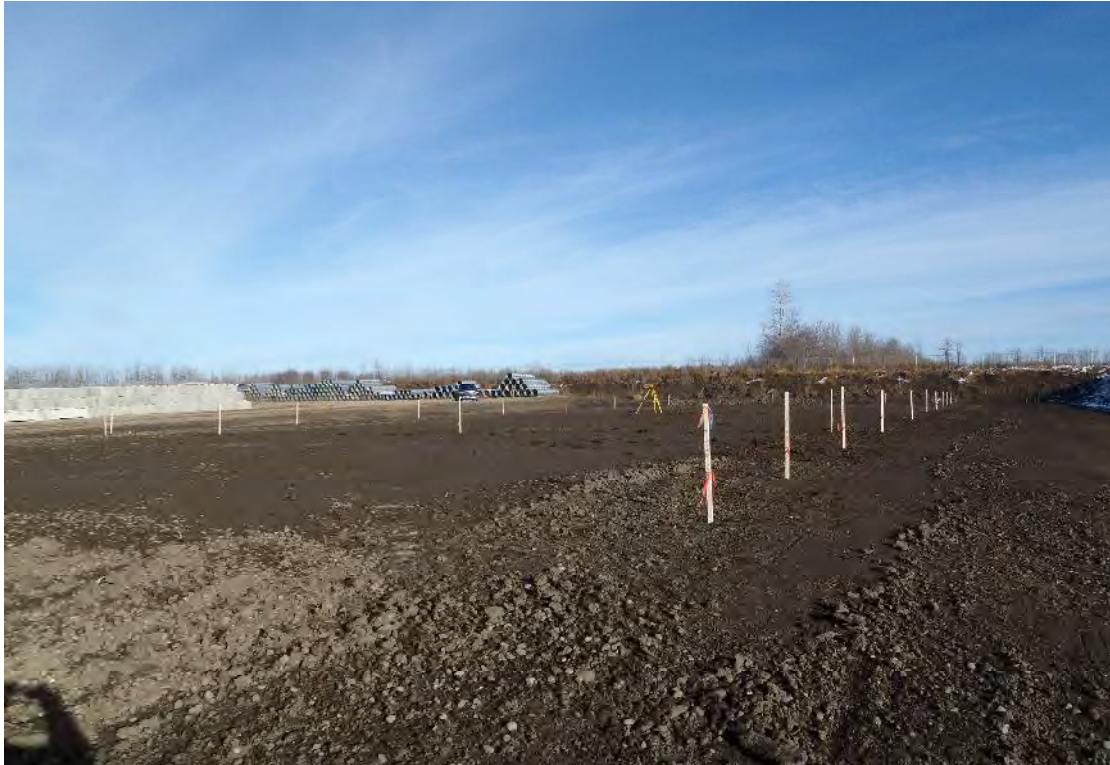
Survey Layout for Granular Base Course - Facing Northeast
