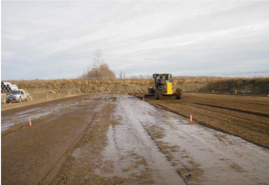
Watering and Compacting Granular Base Course - Facing East
