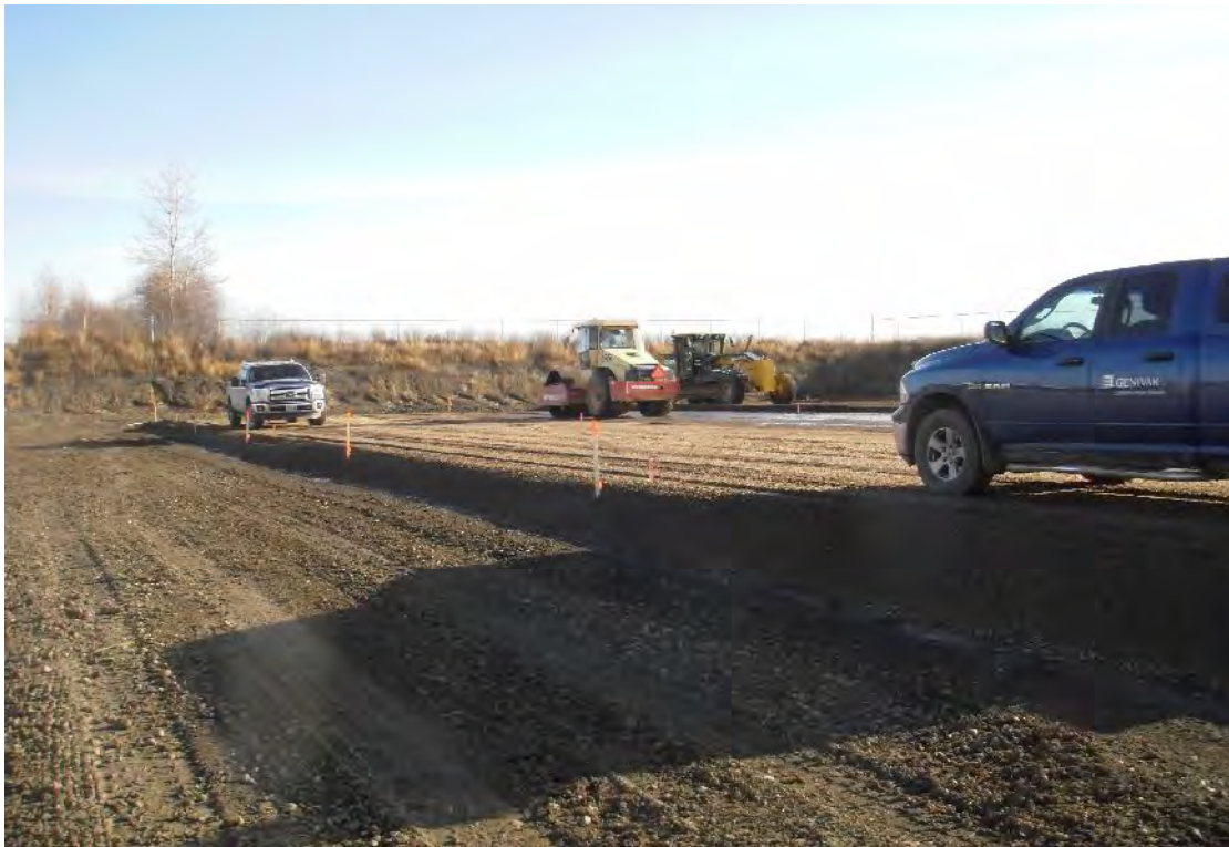
Granular Base Course Installation - Facing East
