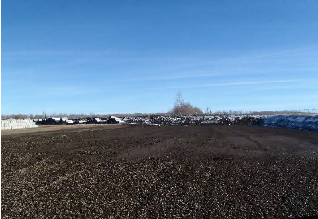
Pad Subgrade Prior to Granular Base - Facing East
