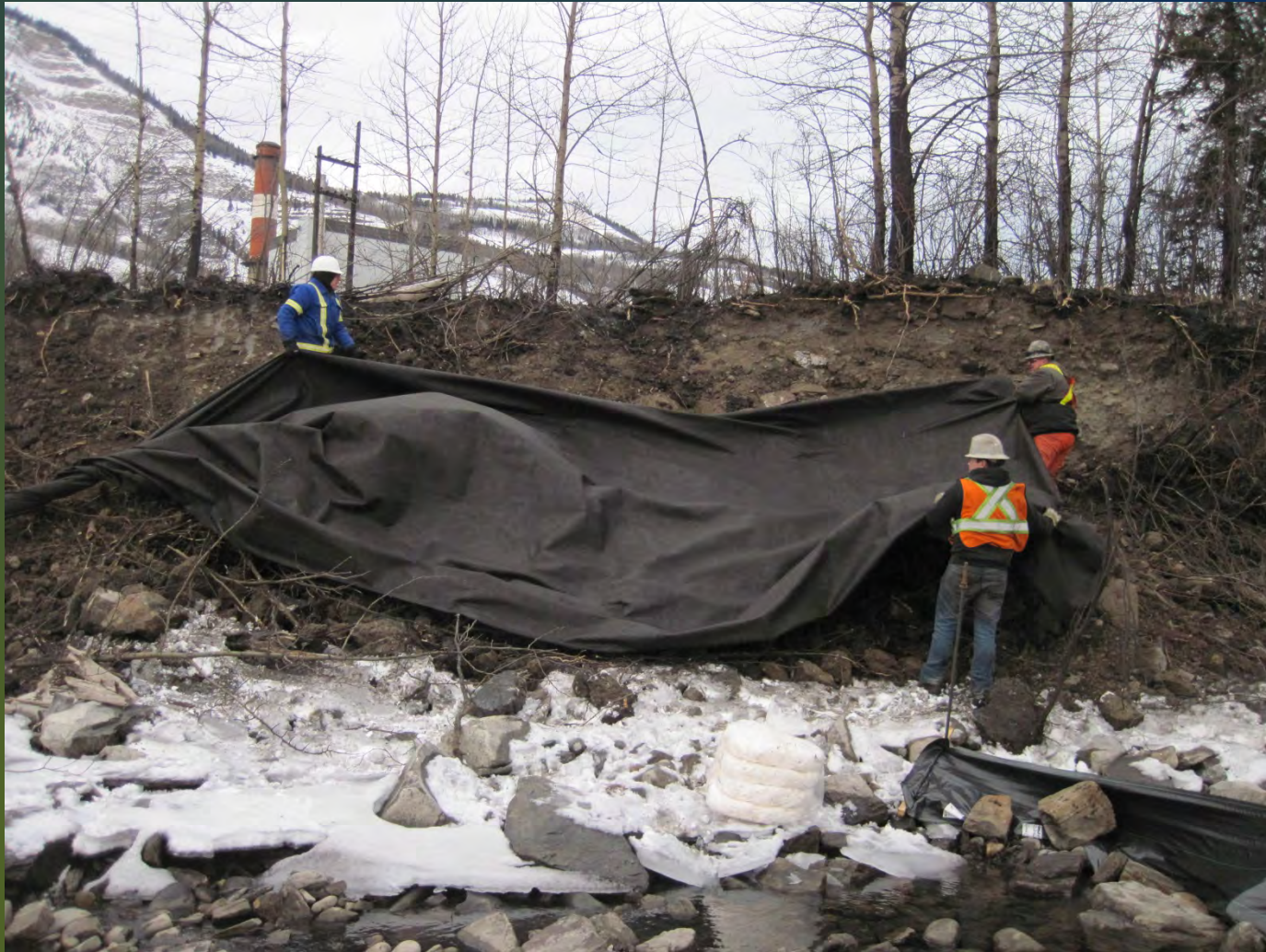
Placing geotextile
