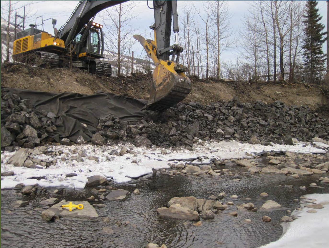
Placing first layer of smaller rock
