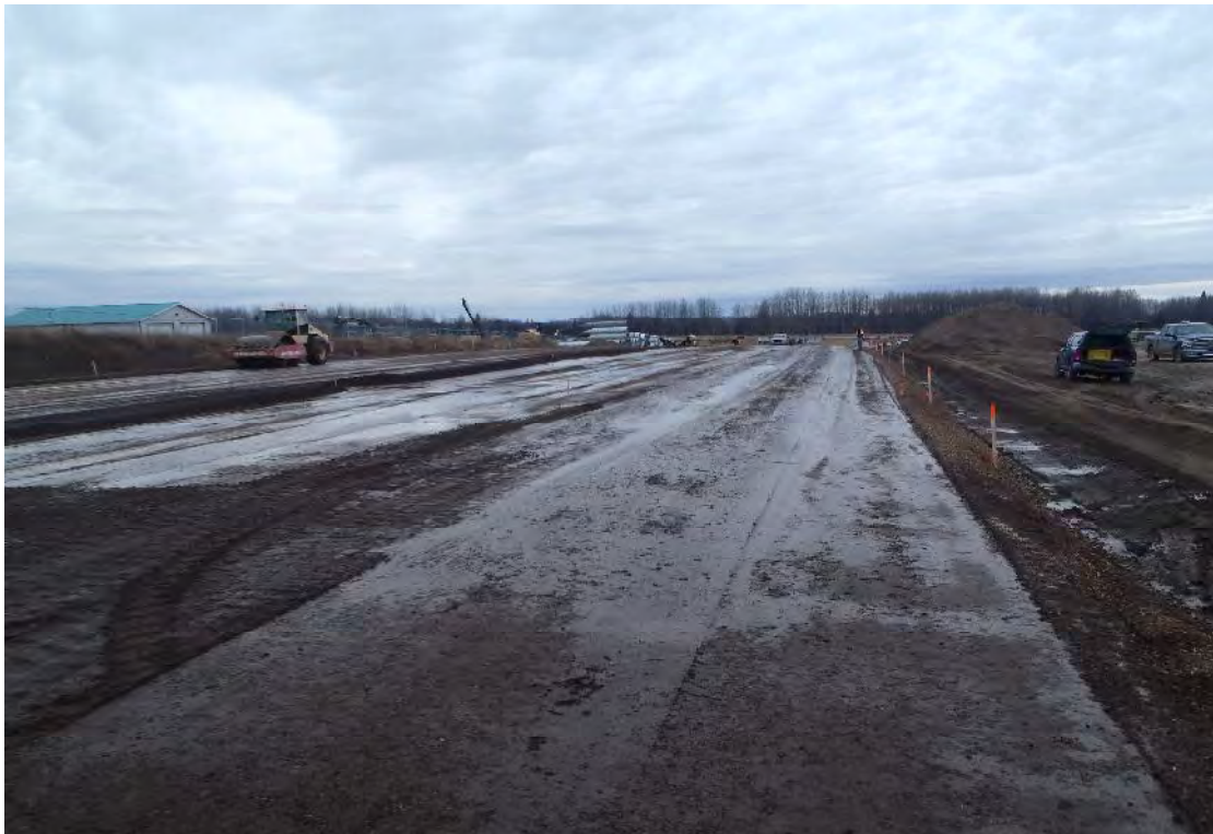
Watering and Compacting Granular Base Course - Facing East
