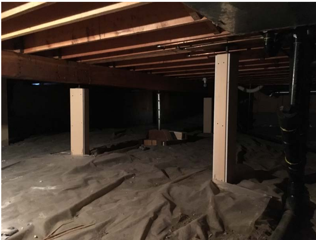
Metal Support posts on concrete sleepers
