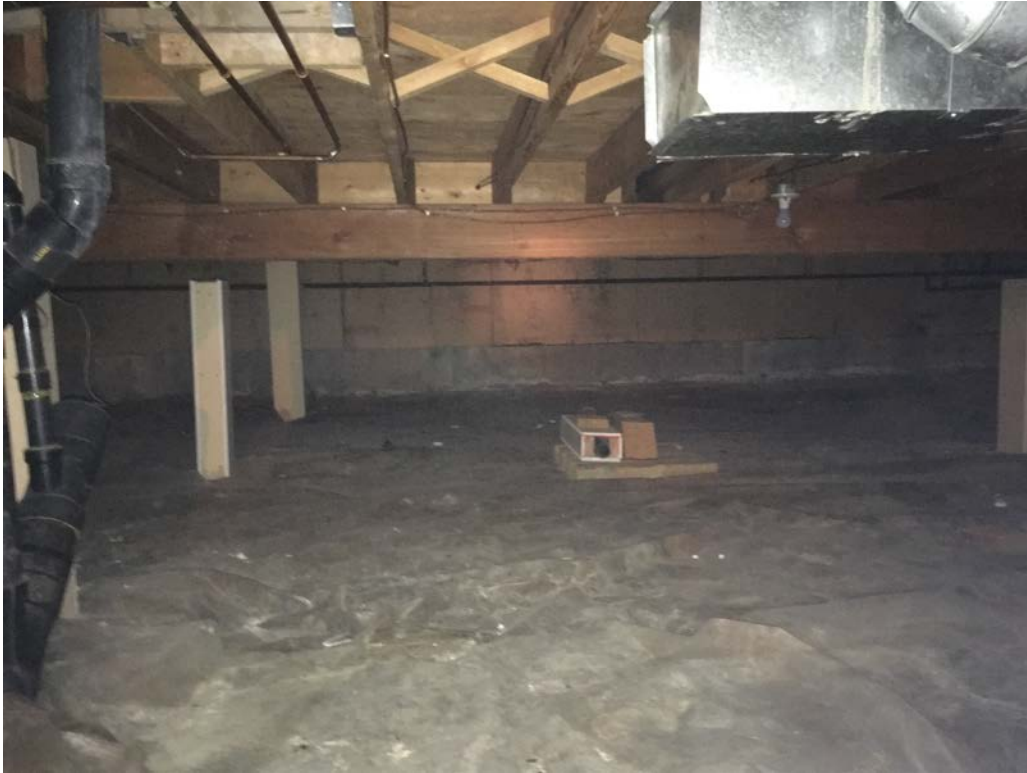
2X8 Floor Joists on 24" centers spanning 13'
