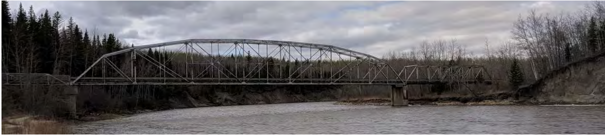
Figure 5: Bridge Elevation Looking West
