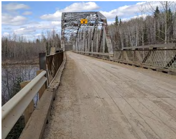
Figure 6: Horizontal Misalignment at Pier 2
