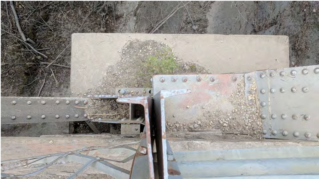
Figure 9: Span 2 and 3 Trusses Jammed at Pier 2
