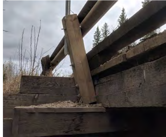
Figure 4: Span 1 Bridge Rail
