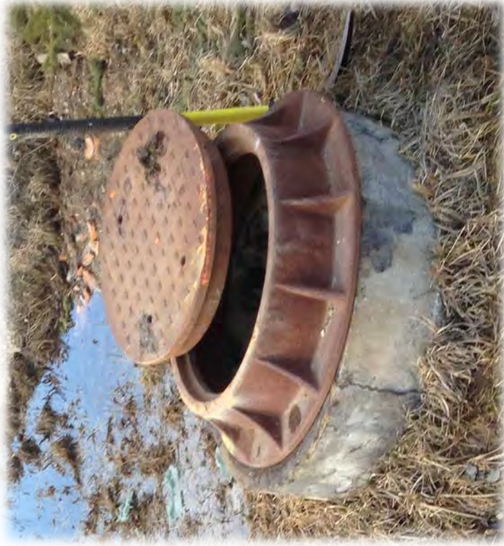
Advanced Trenchless Inc.
