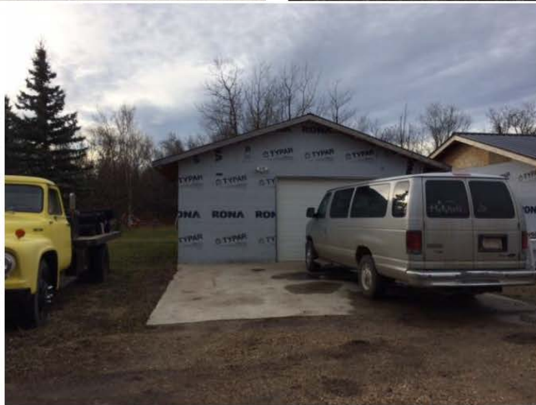
Pic#1 Pin inside Power Pole / Pic #2 – Standing at pin and shooting to north, pole is not directly in line with power pole by pin / Pic #3 – Garage (see distance from tree north of power pole in pic#2)
