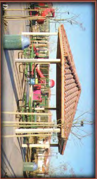
D Neighborhood Park, Las Vegas, NV: This 26' model creates a Southwestern style using a tile roof over a 2" x 6" tongue & groove sub-roof.
